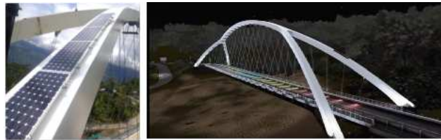
SYSTEM OF PHOTOVOLTAIC SELF SUPPLY LIGHTING -TEQUENDAA BRIDGE (COLOMBIA)
