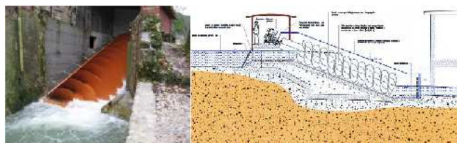
MINIHYDRO PLANT 100%GRID SUPPLY OR STAND-ALONE PLANTS - ITALY
